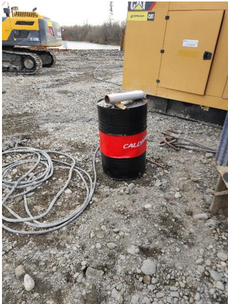
Hazardous material storage on construction site
