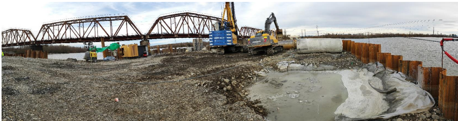
Panoramic view of construction works around the peninsula
